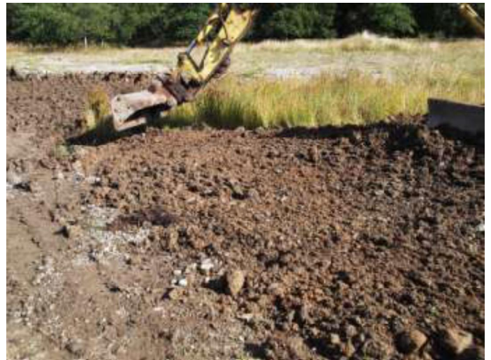
Subsoil being spread
