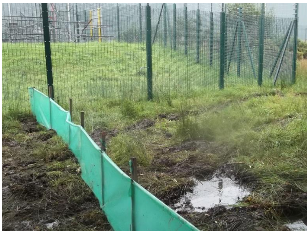
Plate 2: Reptile fence (north eastern end)
